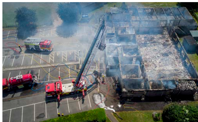
The fire at Bromham Social Centre in June 2021.
