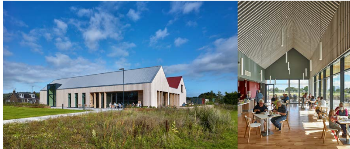
The Larick Centre, Fife by Collective Architecture
