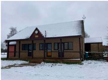
The existing sports pavilion
